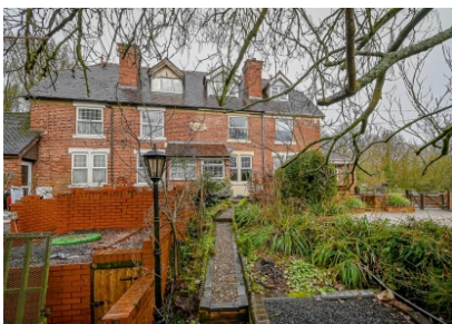
3 The Elms, Station Road, Highley, Bridgnorth
