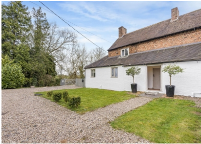
Blythbury Farmhouse Cottage, Shifnal
