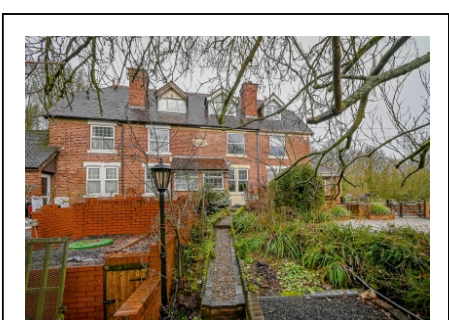
3 The Elms, Station Road, Highley, Bridgnorth
