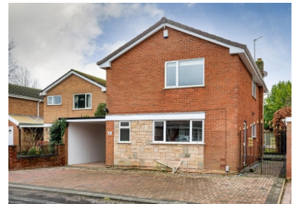
21 Bellencroft Gardens, Merry Hill, Wolverhampton
